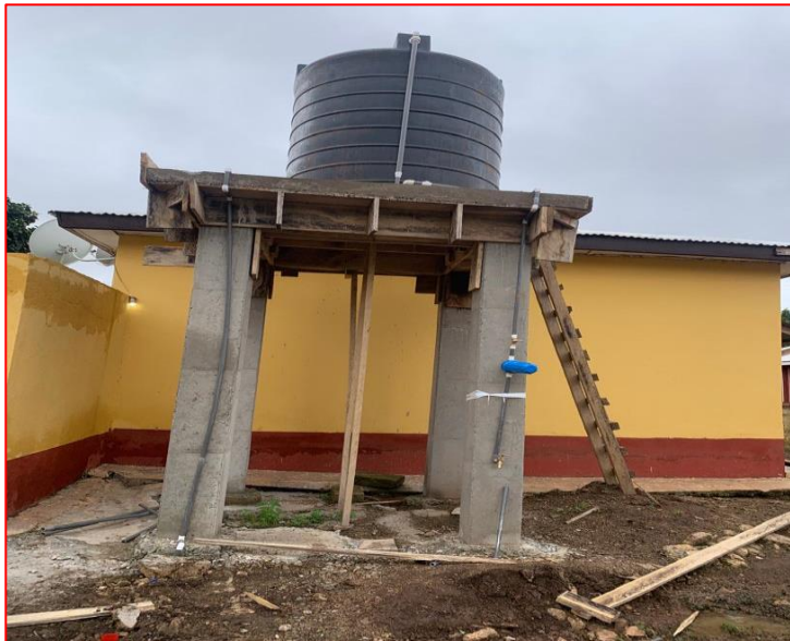
Drilled and mechanized of 1no. Borehole at Berekum college of Education
