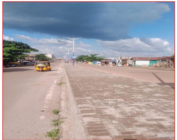
Street Lights and Pavements Constructed at Various Locations
