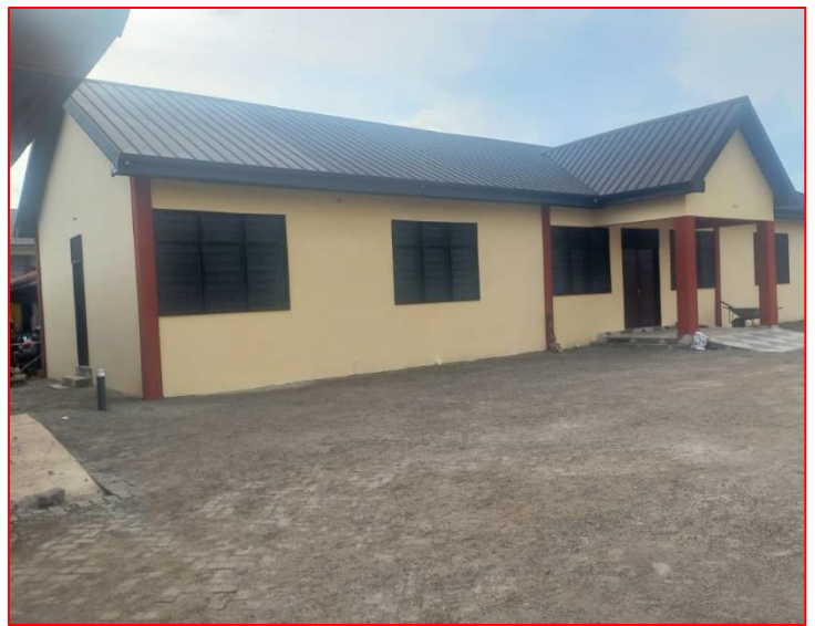
Completed 1no. Meat shop at Berekum Thursday Market
