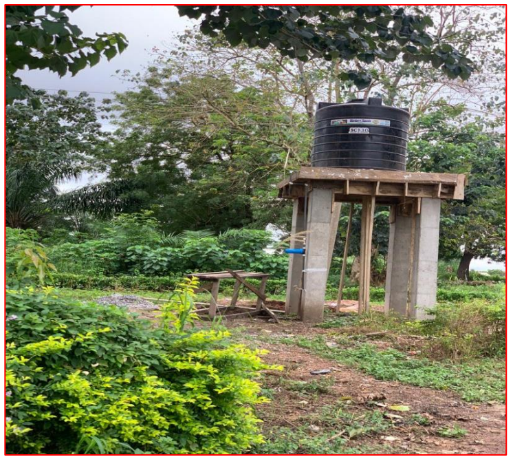
Drilled and mechanized of 1no. Borehole Continental
