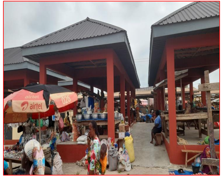
Completed 2no. Pavilion and paving of market access and market spaces at Berekum
