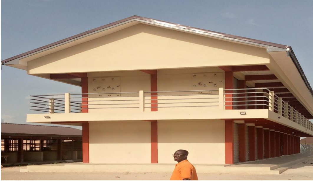
Completed 2 storey 48 unit Lockable stores and external works at Berekum Thursday Market (GSCSP)
