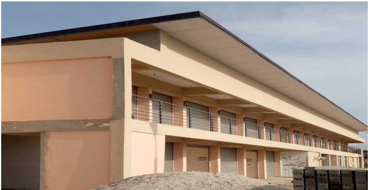
Completed 2 storey 40 unit Lockable stores, banking hall and external works at Berekum Thursday Market (GSCSP)
