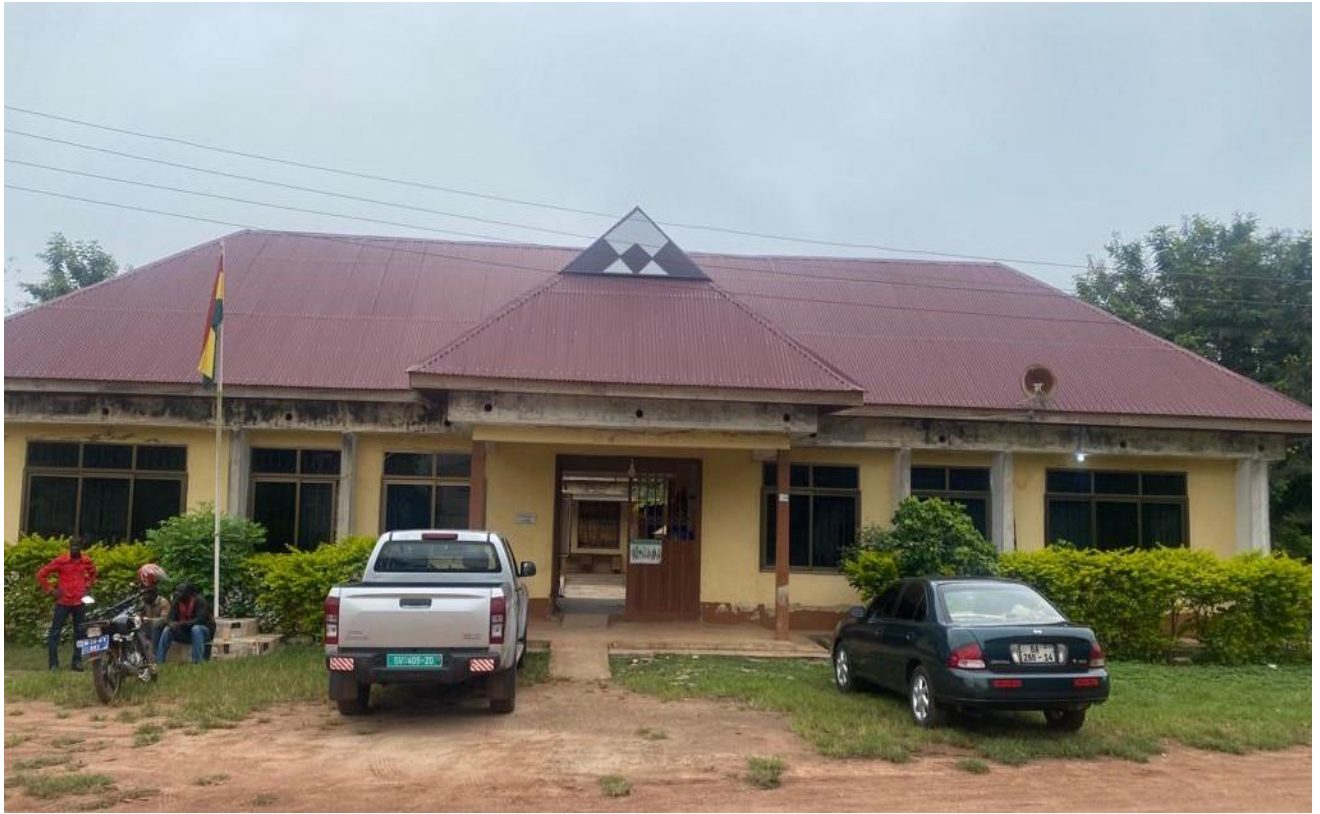
(Renovation of GES office block) - - DACF
