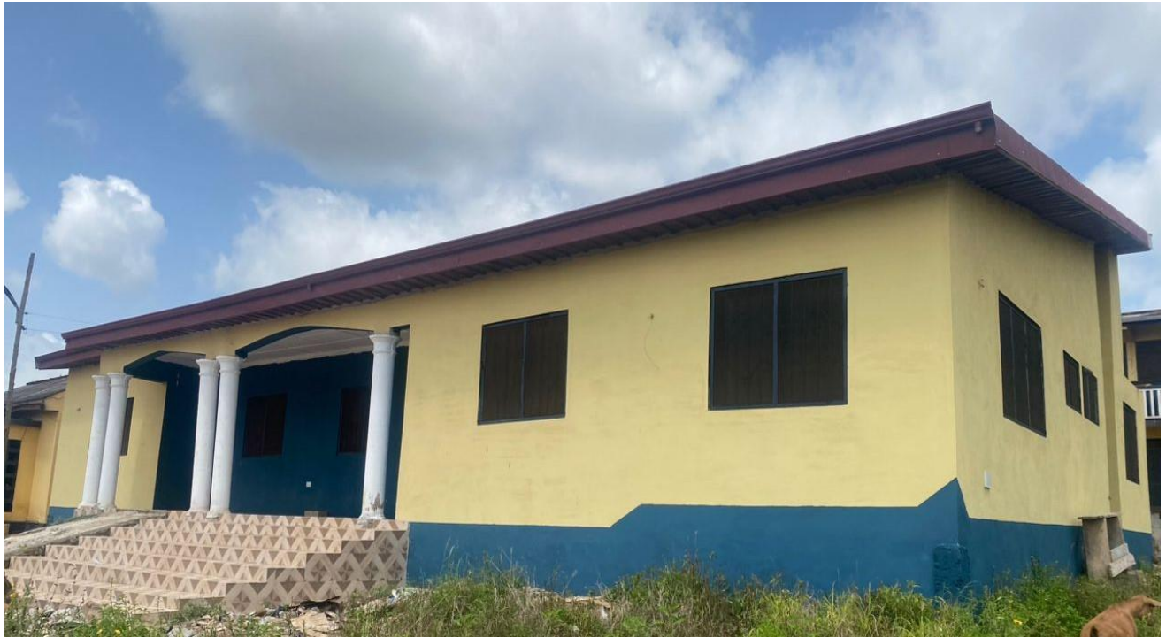
(Completed Police Station at Berekum Charge Office) – DACF-RFG
