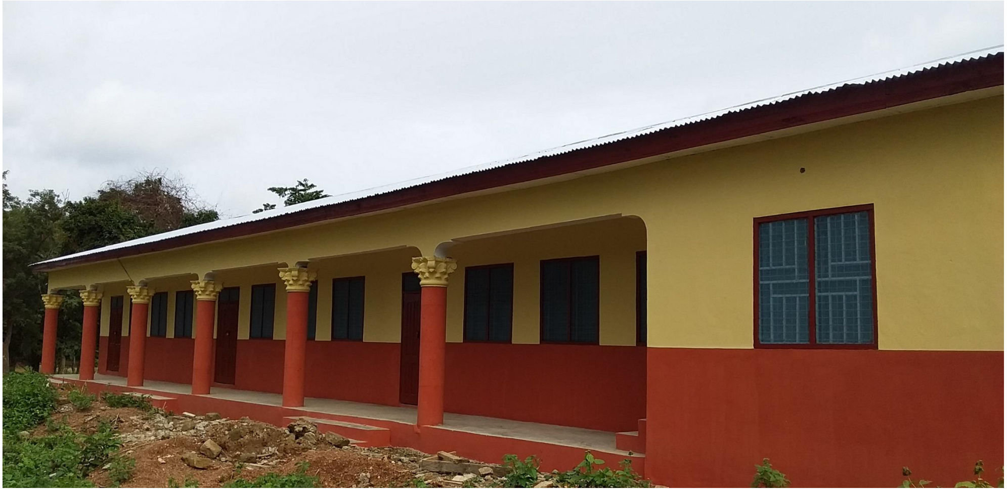
Figure 6. Construction of iNo. 3-Unit Classroom Block with ancillary facilities at Anyinasu
