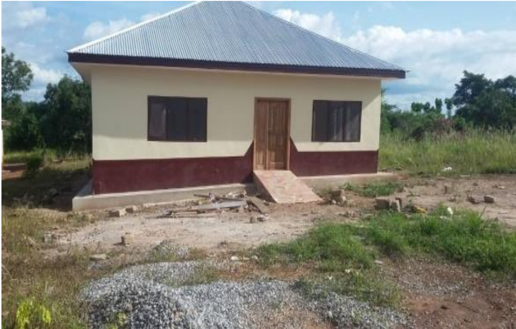
Figure 5. Completion of CHPs Compound with supply of basic equipments at Oforikrom
