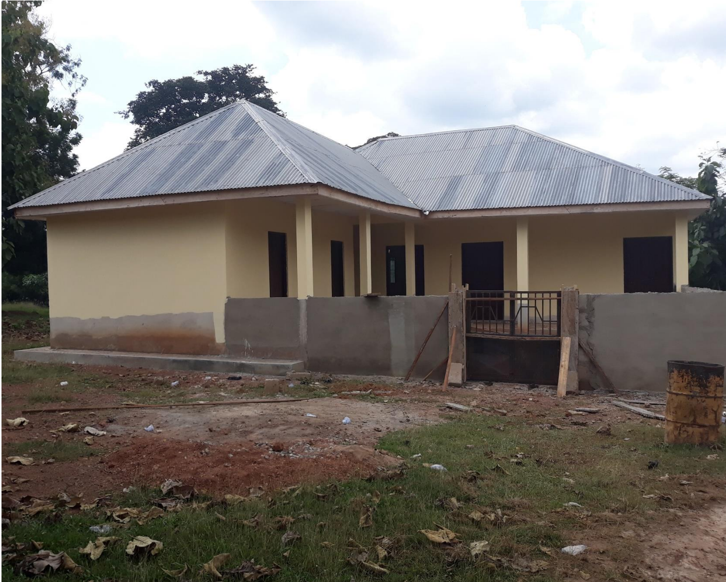
Figure 2 Construction of 2-Unit KG School Block with ancillary facilities at Akorofo
